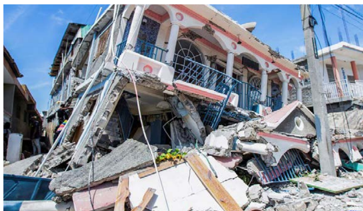
The earthquake caused significant damage to property and infrastructure
